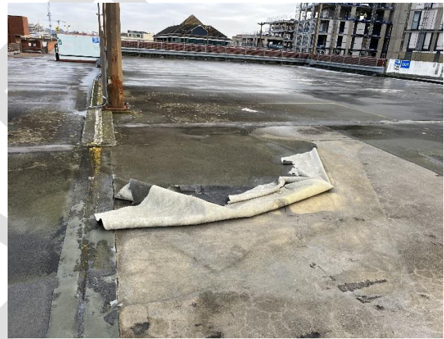
Fig. 12 – Damaged waterproofing
