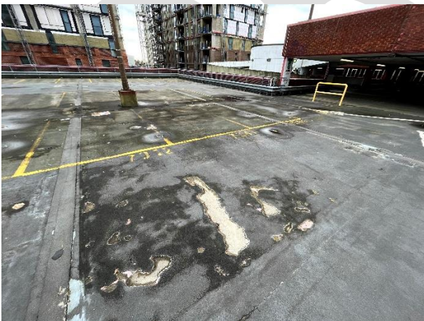
Fig. 13 – Damaged waterproofing
