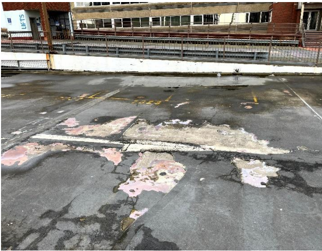
Fig. 11 – Damaged waterproofing
